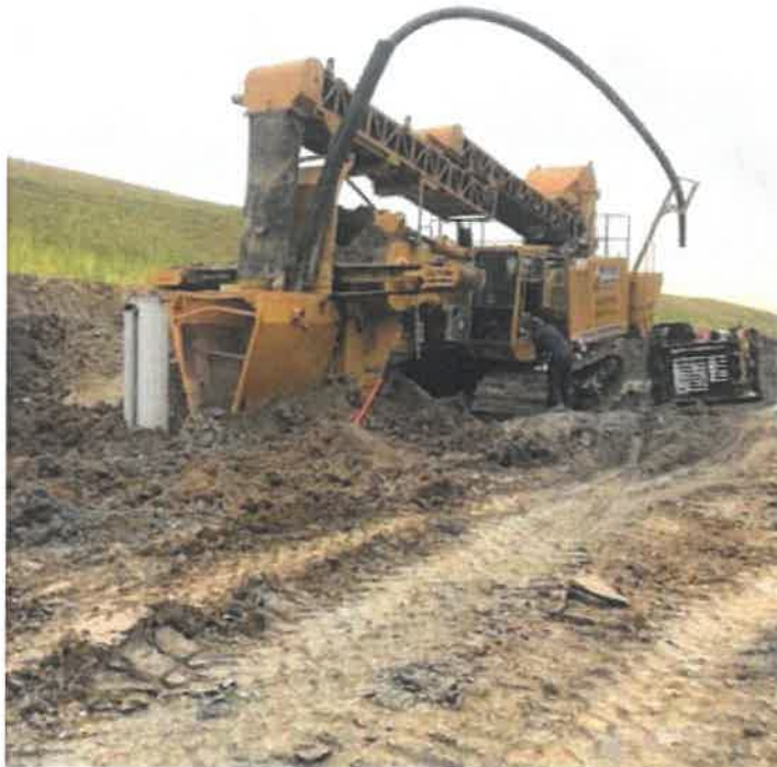
Photo 2: Installation of the Deep Seep Collection Trench in October 2019.
