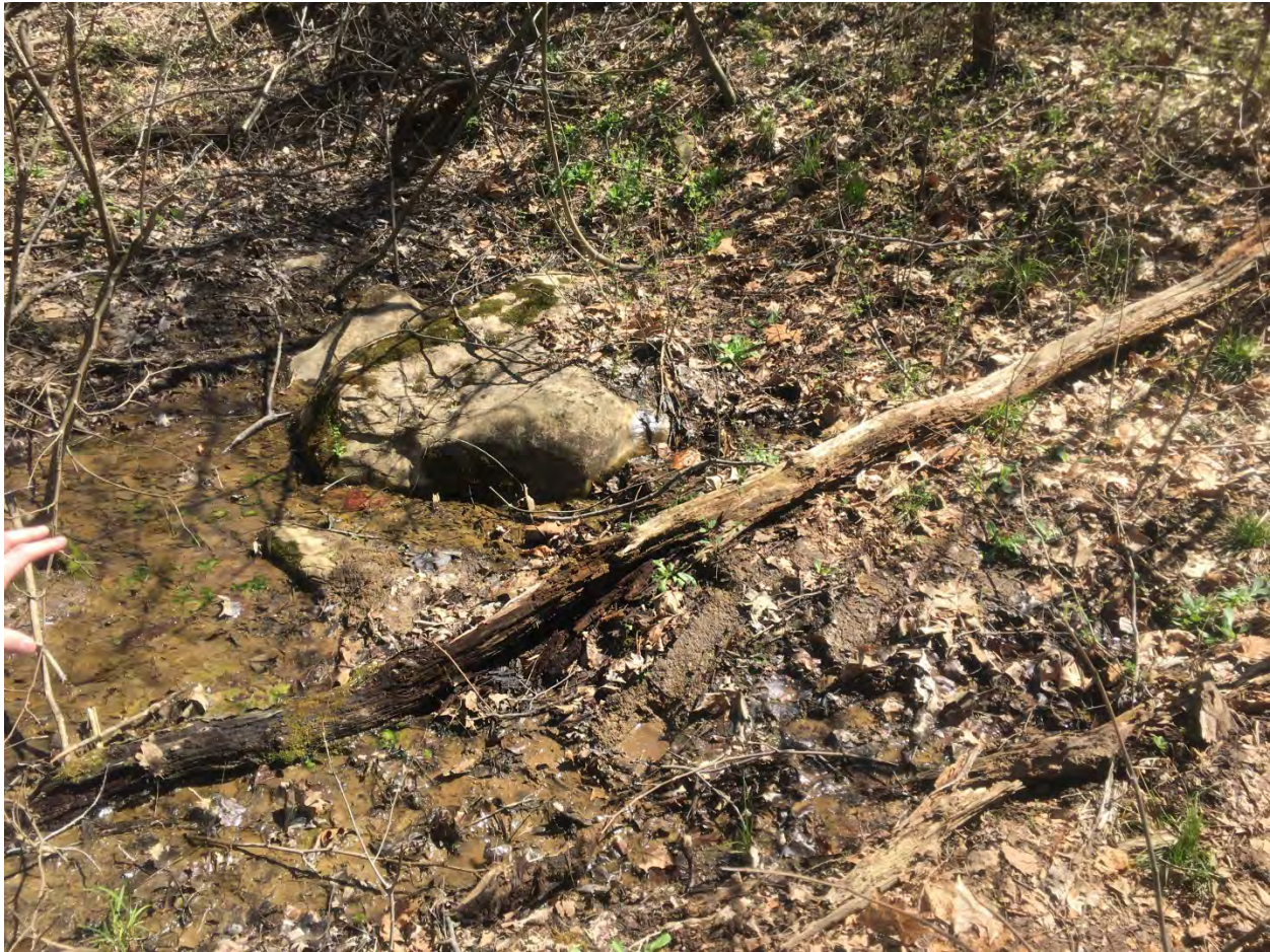
Photo 1: The NW Seep as observed on April 9, 2019.
