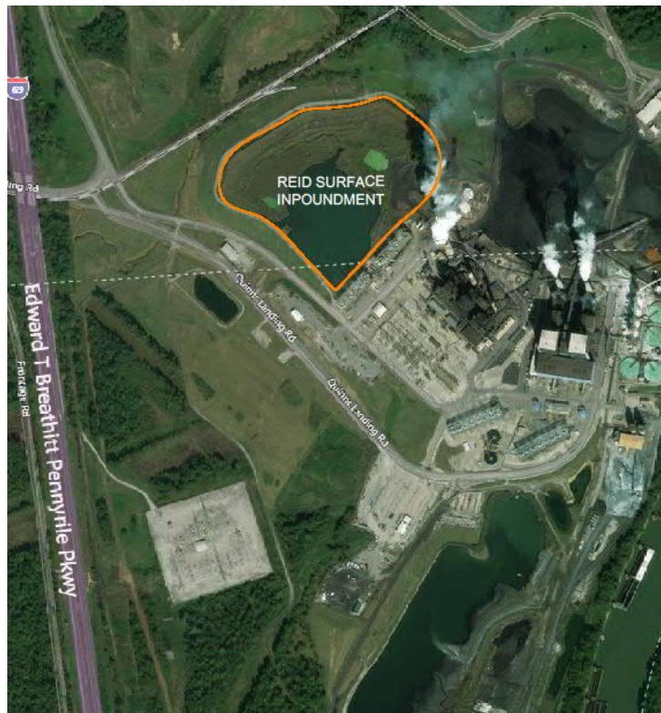
Figure 2: BREC Reid/HMPL Surface Impoundment Site Location
