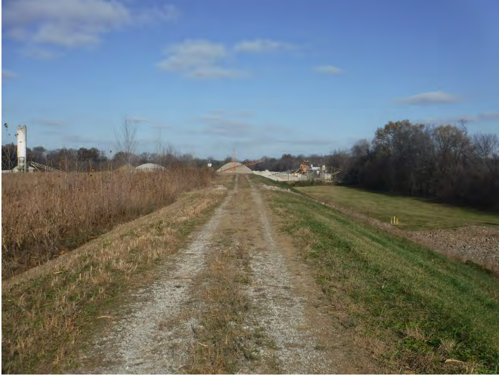
1 – Top of Dam – East Leg
