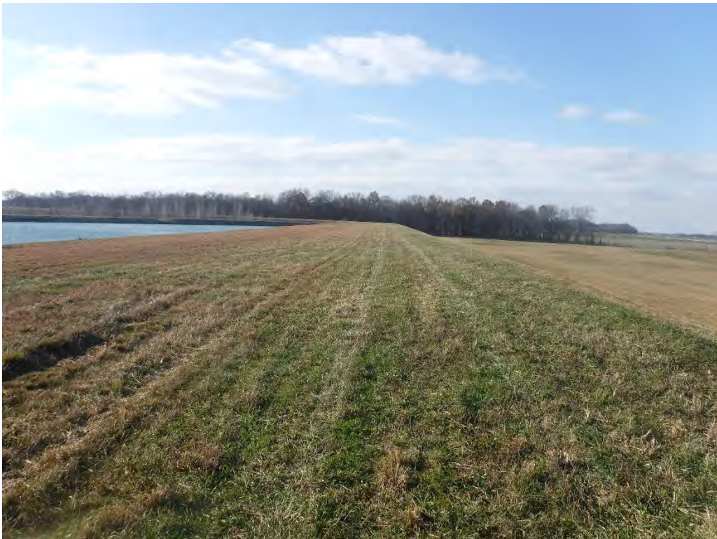
14 -- Top of Dam – NW Leg
