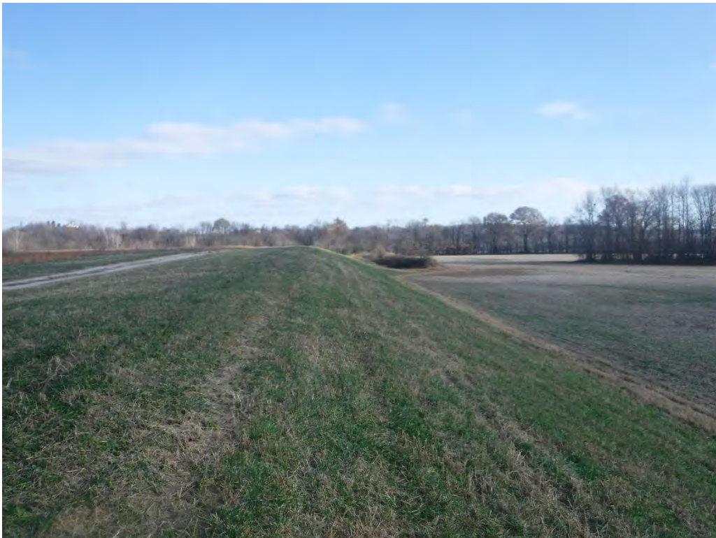
2 – Downstream Slope – SE Leg
