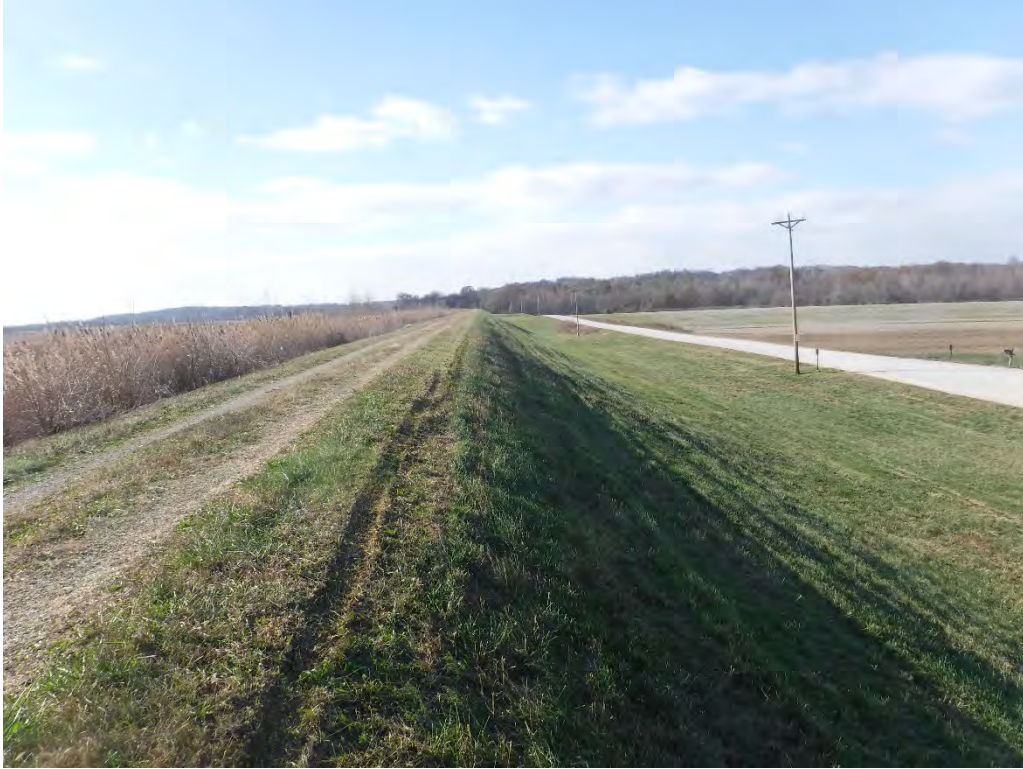
9 – Downstream Slope – North Leg
