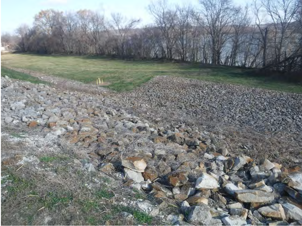
7 – Downstream Slope @ Spillway
