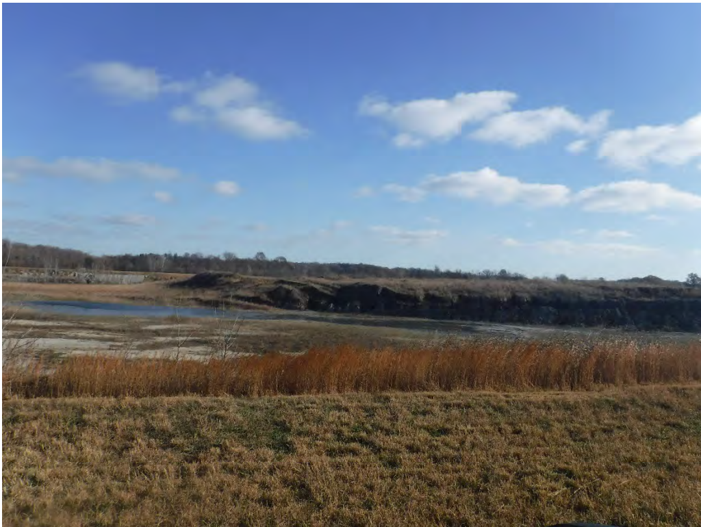
8 – General – Upstream View
