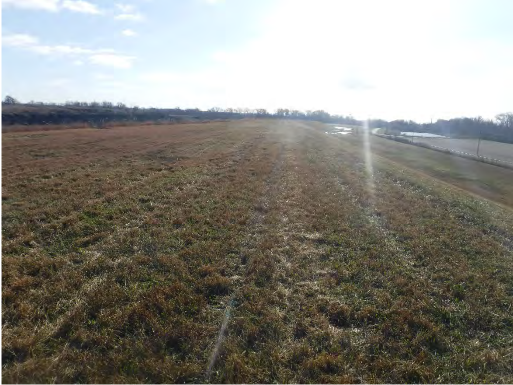
17 – Top of Dam – SW Leg
