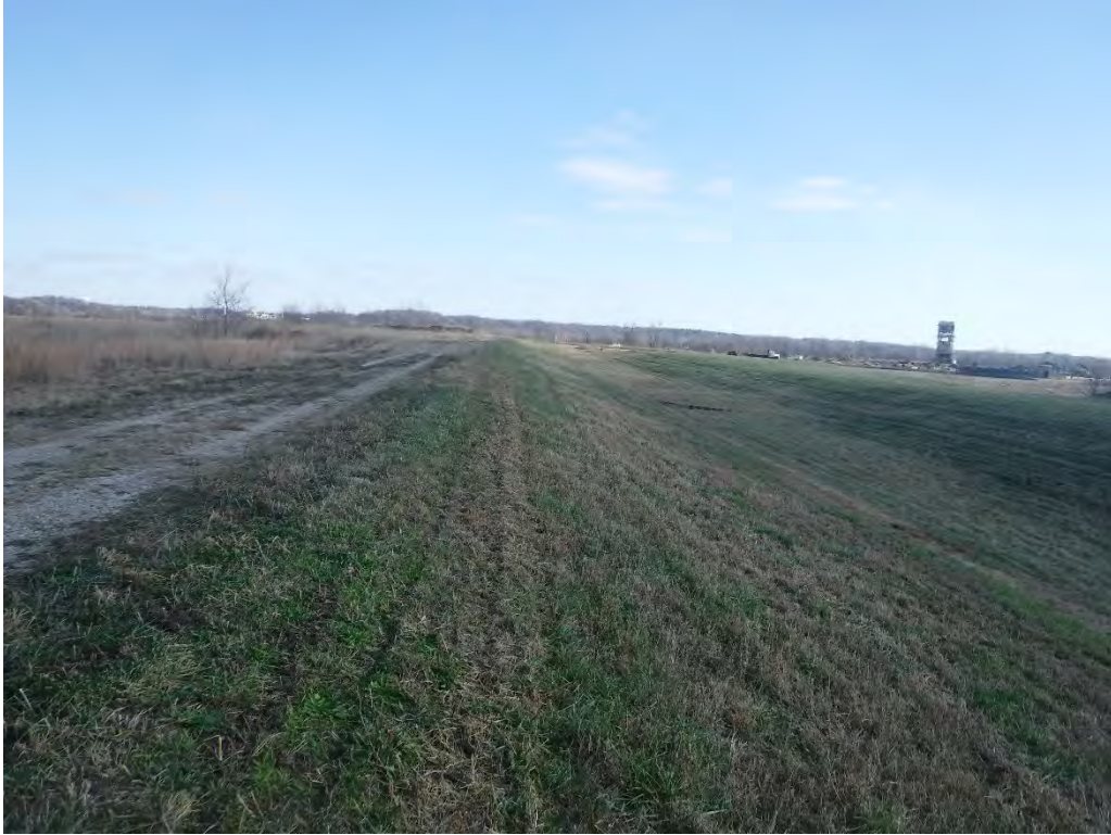
15 – Downstream Slope – South Leg
