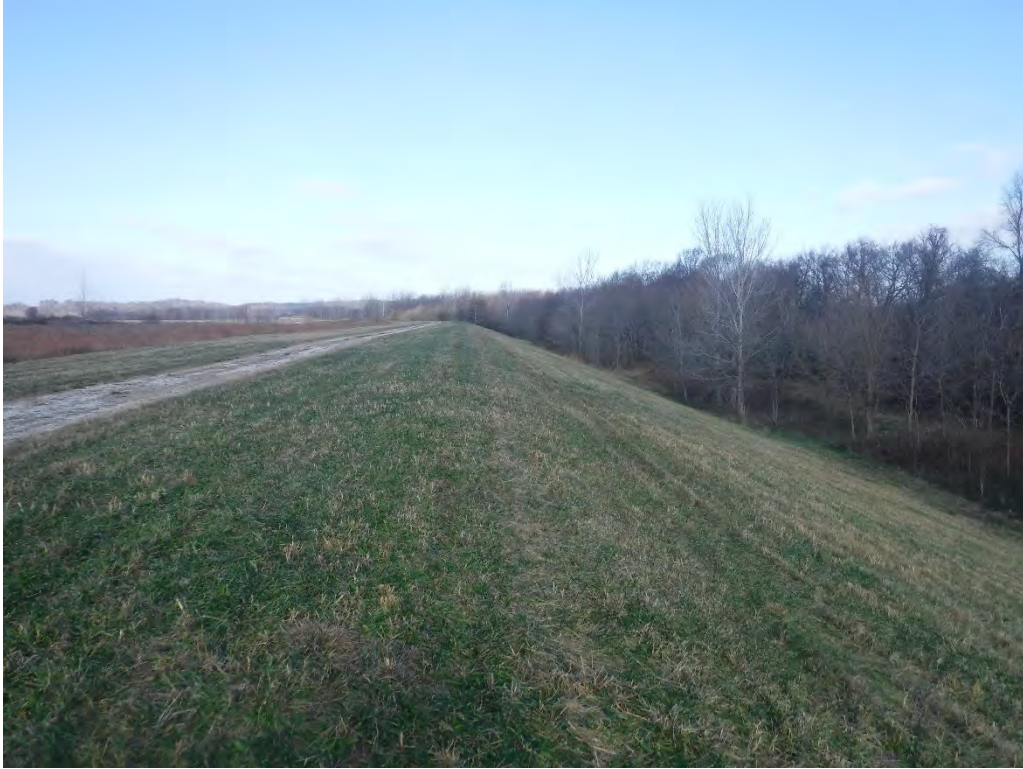
5 – Downstream Slope – NE Leg
