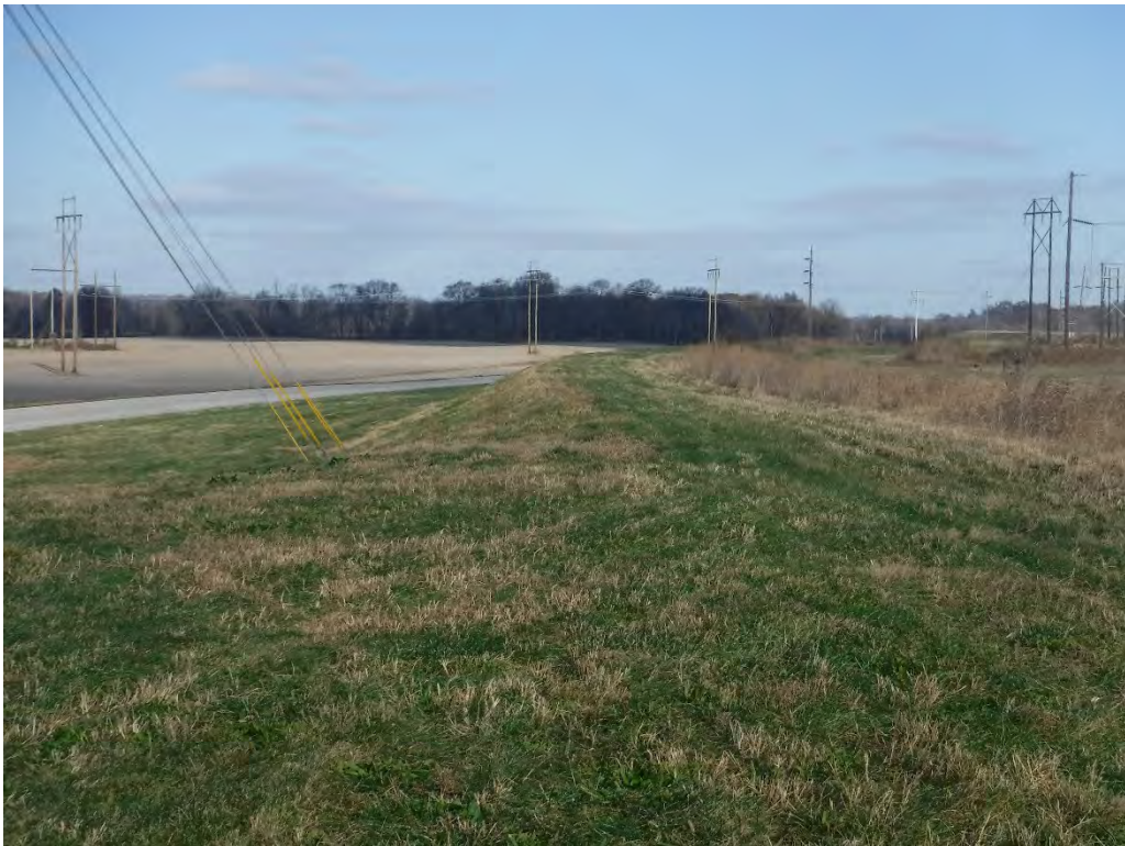
6 – Top of Dam – West leg
