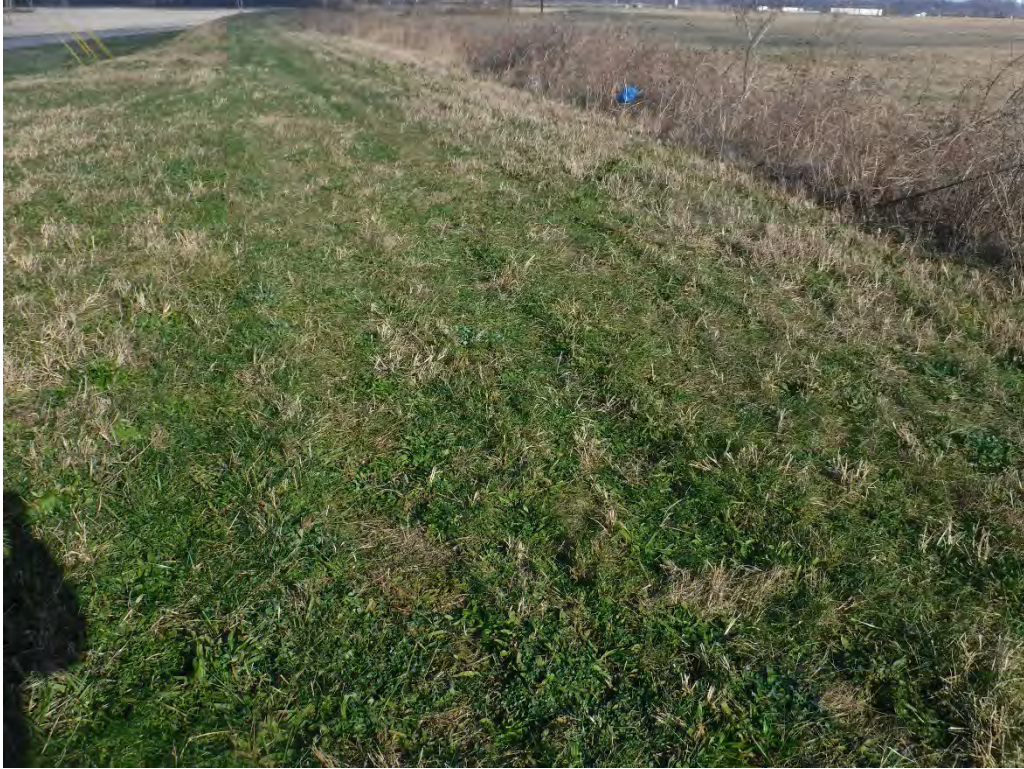
7 – Upstream Slope – West Leg
