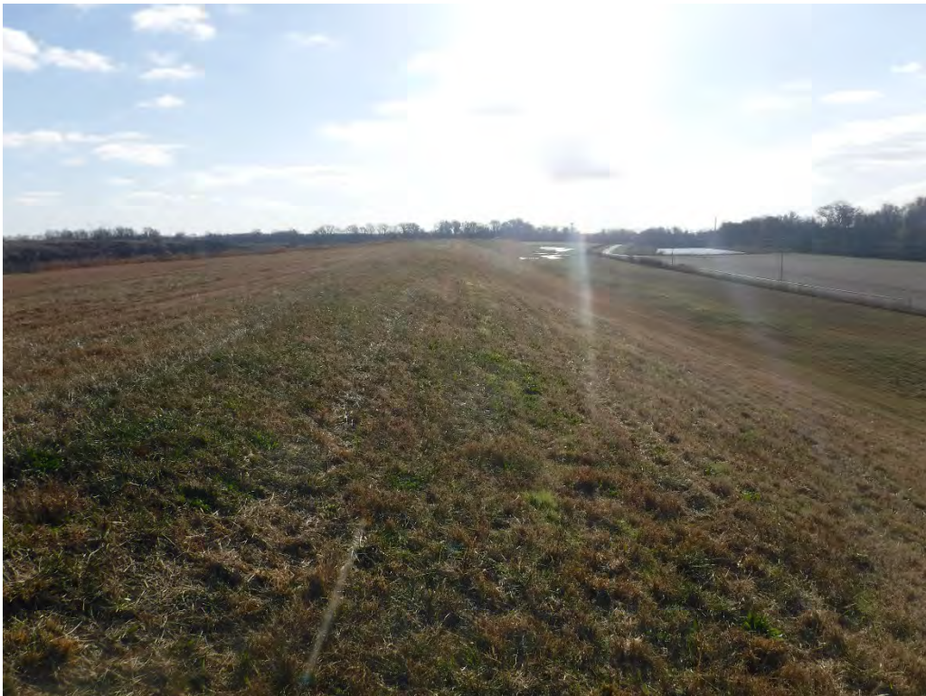
18 – Downstream Slope – SW Leg
