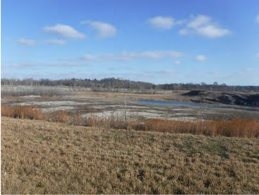
7 – General – Upstream View
