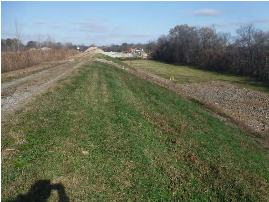
2 – Downstream Slope – East Leg
