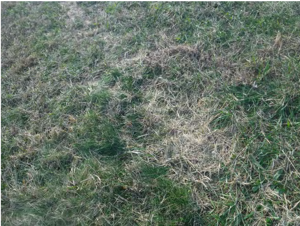
6 – Rutting from Mowing Downstream Slope
