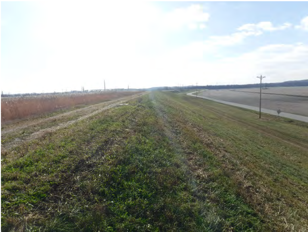
12 – Downstream Slope – West Leg
