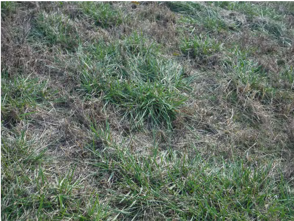
16 – Erosion Downstream Slope
