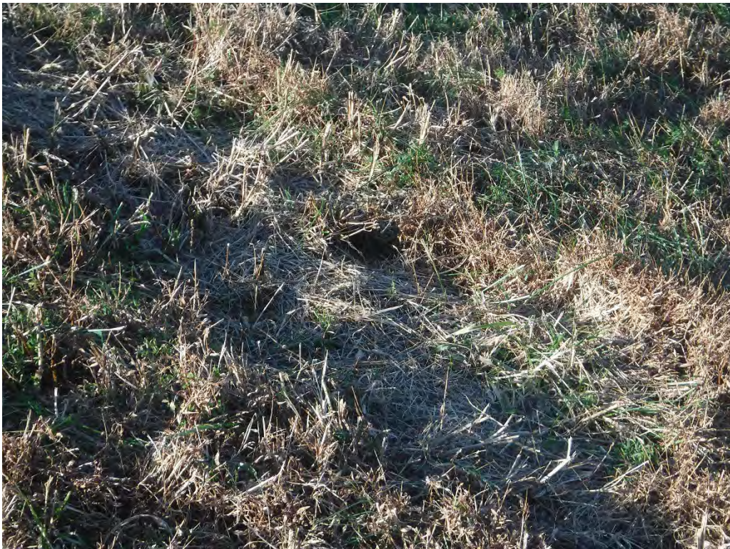
16 – Erosion Downstream Slope
