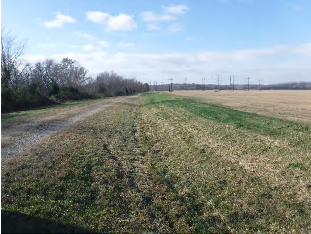
3 – Top of Dam – South Leg
