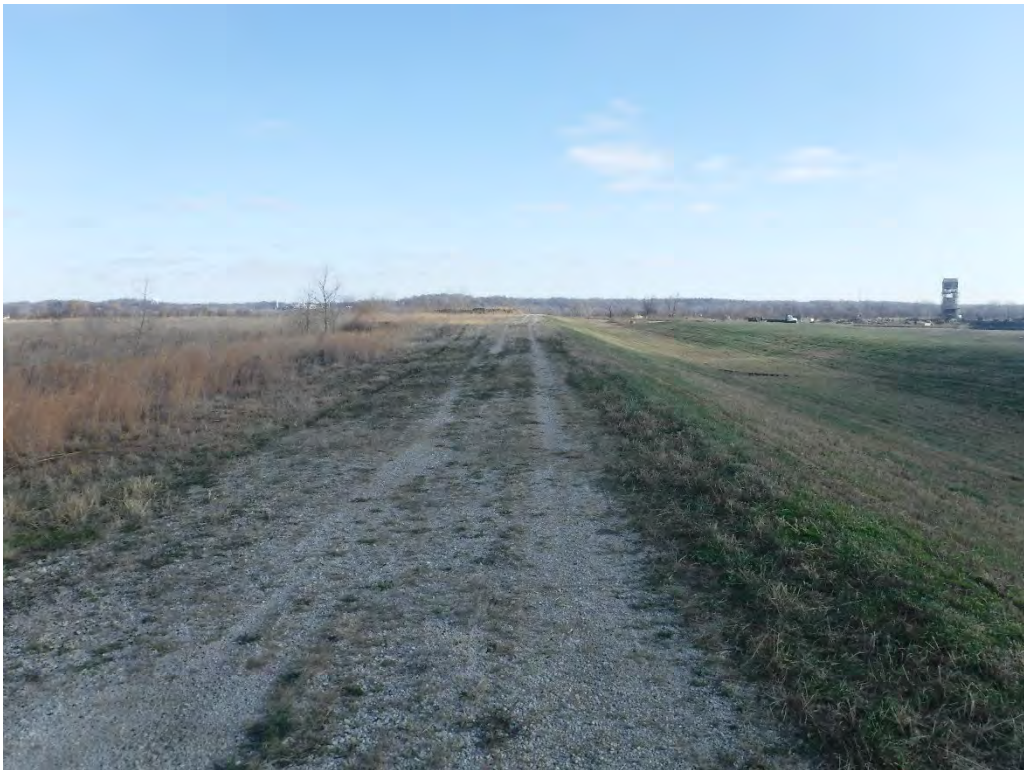
14 – Top of Dam – South Leg
