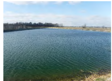
Waste Water Treatment Facility
