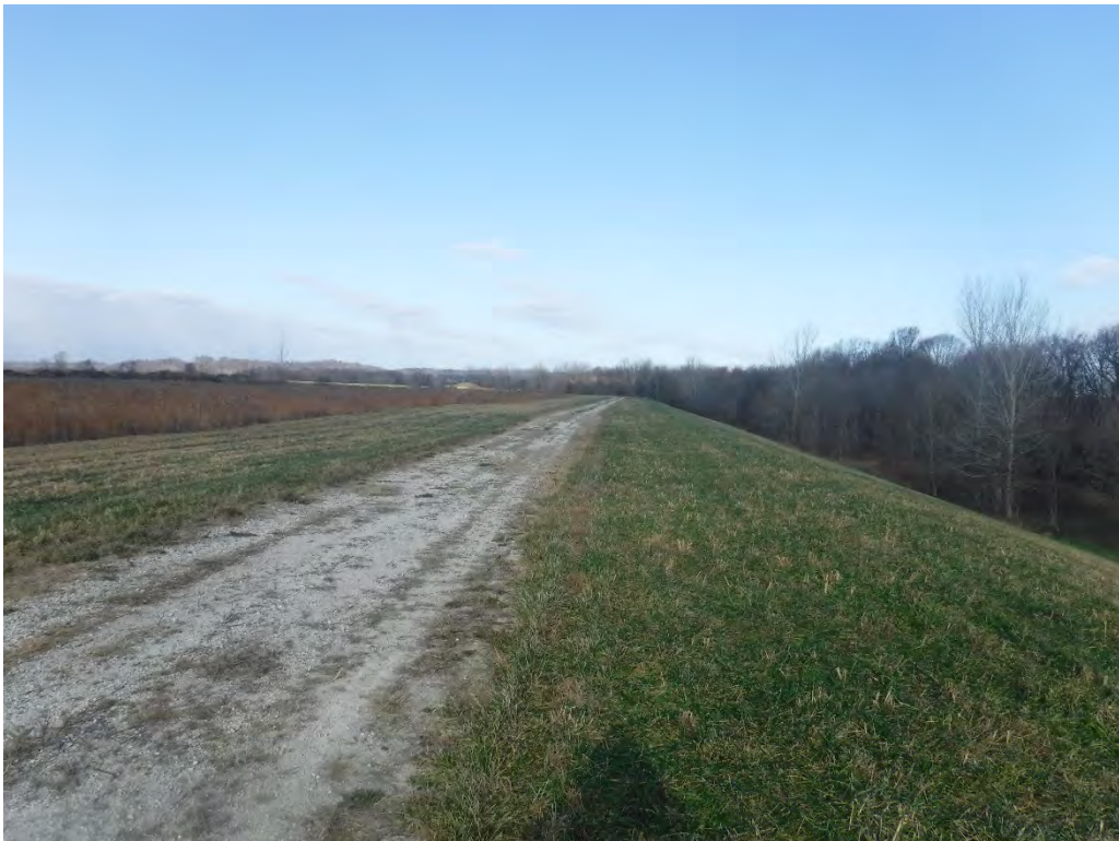
4 – Top of Dam – NE Leg
