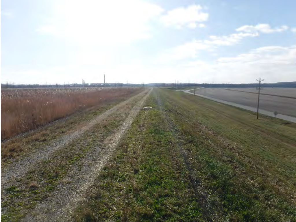
11 – Top of Dam – West Leg
