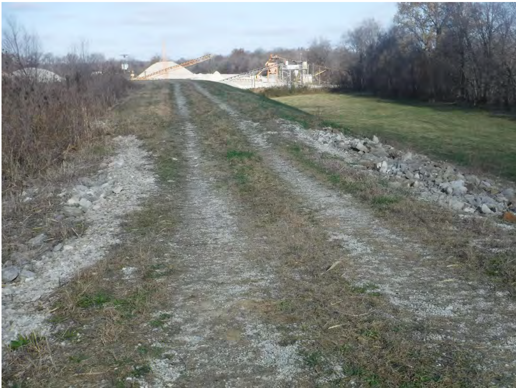
6 – Top of Dam @ Spillway
