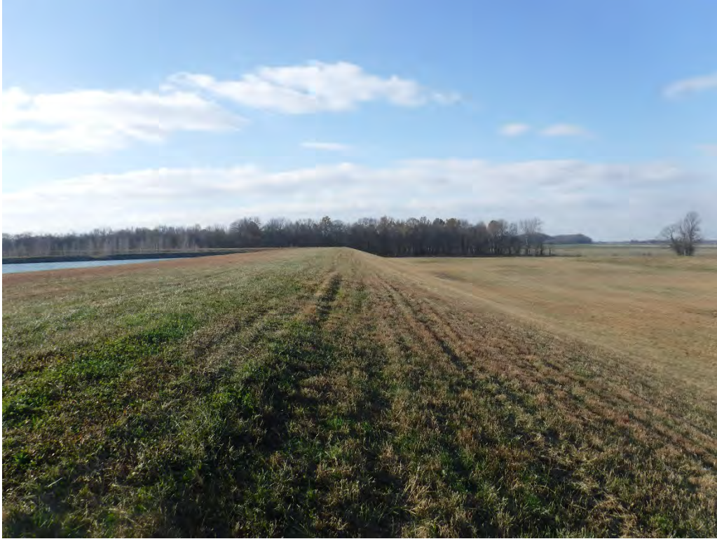
15 – Downstream Slope – NW Leg
