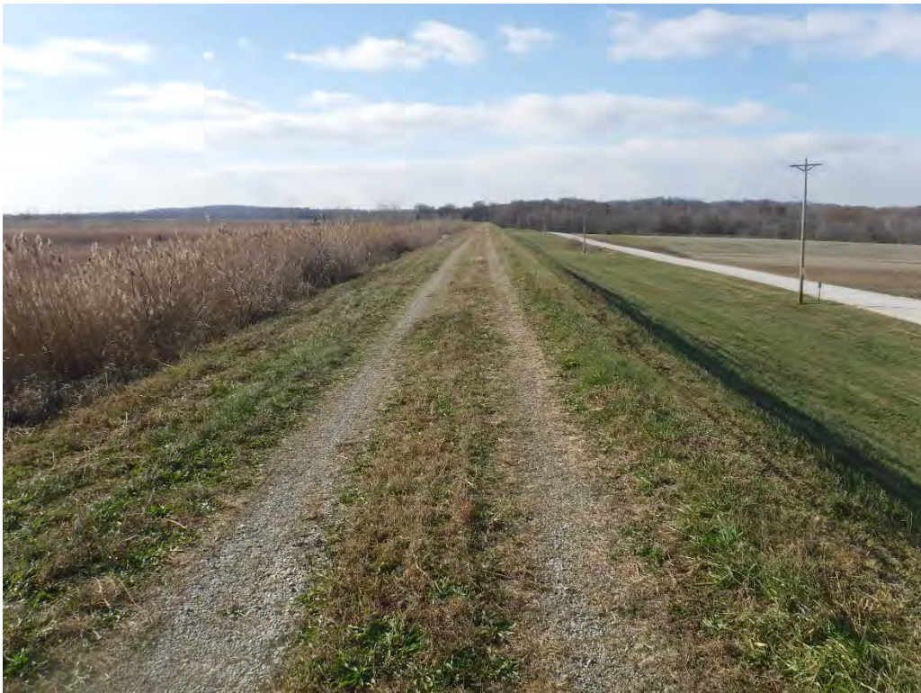
8 – Top of Dam – North Leg
